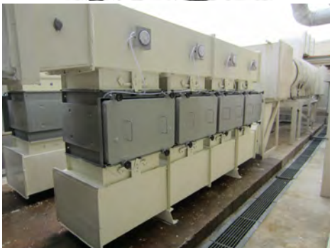
Multi banks BIBO housing connections for higher airflow
